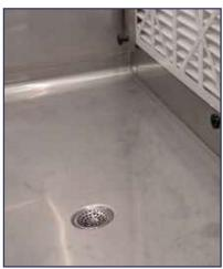
Each **dinovi** air handling unit is composed of washdown chambers made of 304/316 stainless steel. Each unit comes with hygienic certification in accordance with DIN 1946 Part 4:2008.
